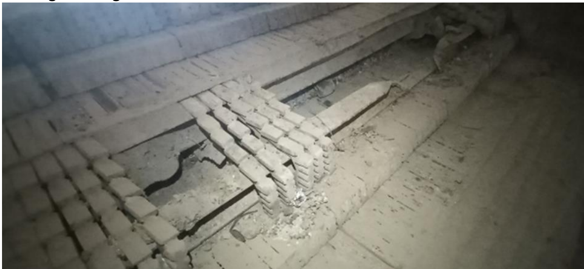
- damage on the grate :
