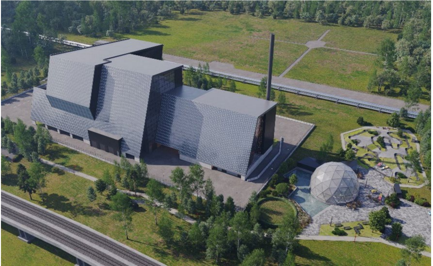
Visual representation of the planned waste-to-energy plant in Latvia © LASUA
